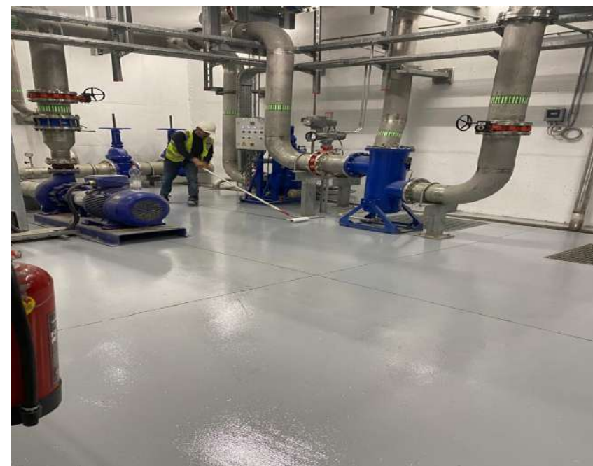
HIDROPOWER STATION Pavafloor 2 System - Thick Film coating
